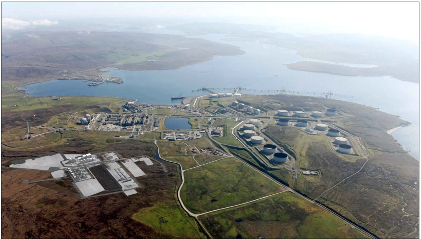
Figure 16 Shetland Gas Project, Scotland, UK (photo: Hauraton)
