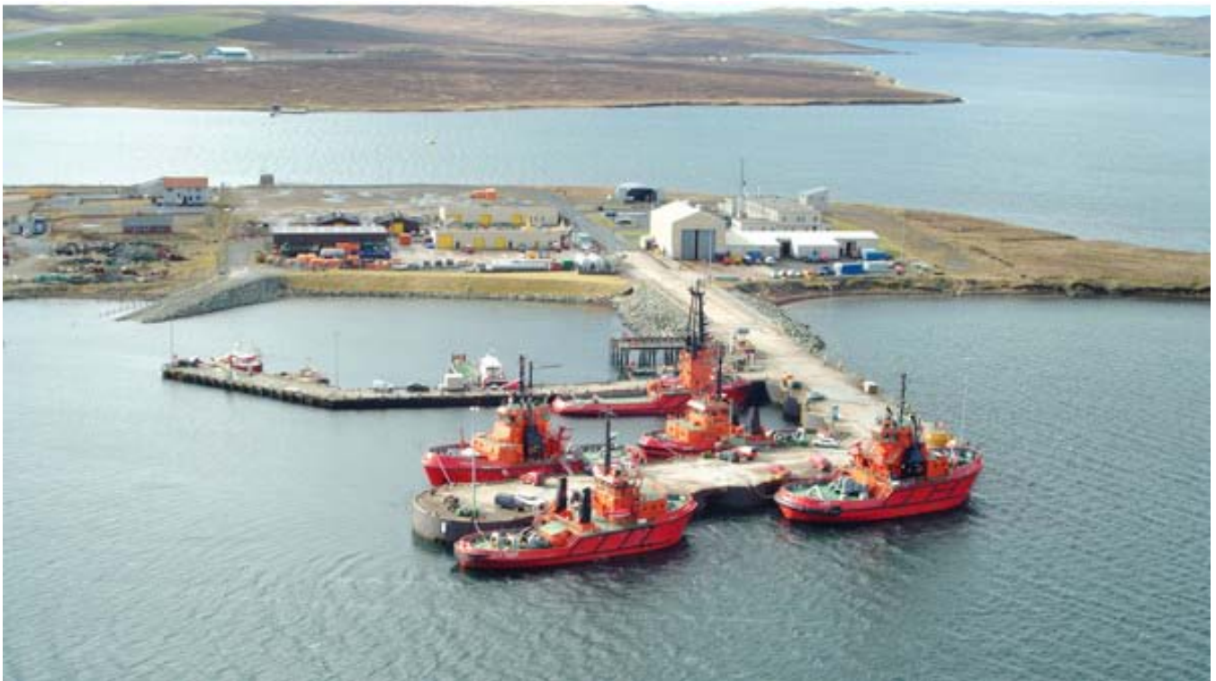
Figure 19 Small jetty for deepwater vessels servicing off-shore fields but which might suffice to supplement a ferry terminal during development of Anticosti oil and gas field (photo: Financial Post, 8 February 2016)
