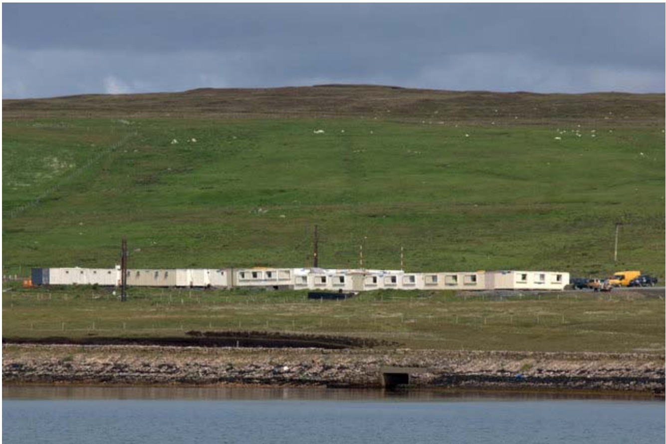
Figure 21 Temporary construction camp (photo: http://www.geograph.org.uk/photo/2466872 )
