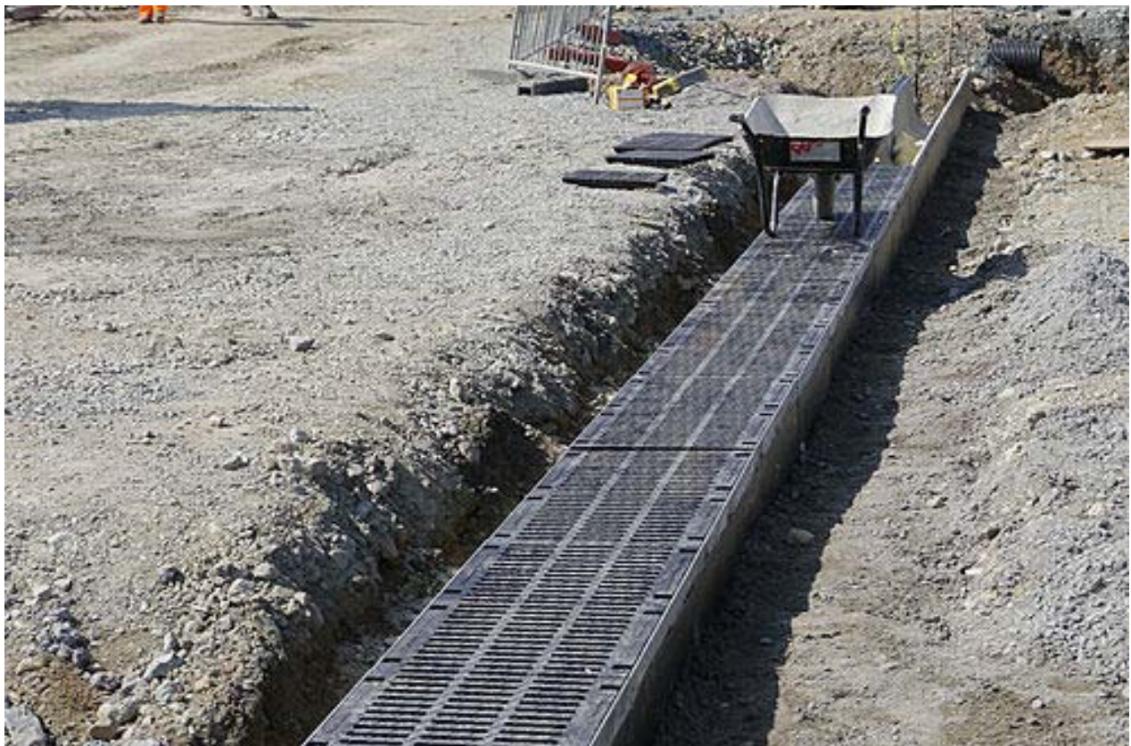
Figure 17 Surface drainage system being installed (photo: Hauraton)
