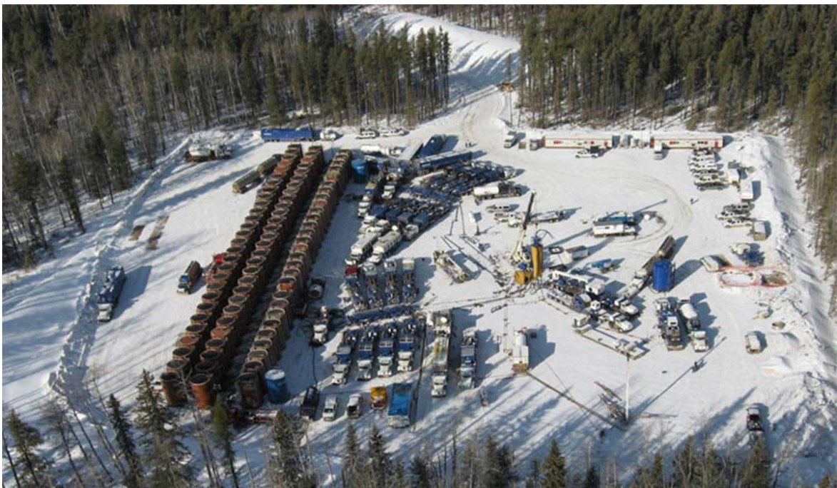
Figure 13 Well pad for hydraulic fracturing in Northwestern Alberta (Trican Industries)
