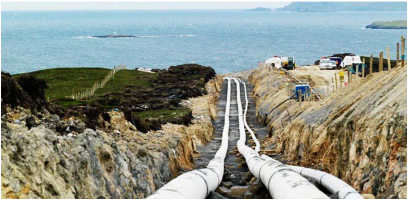
Figure 18 Pipeline construction, Shetland Gas Project (photo: Total)
