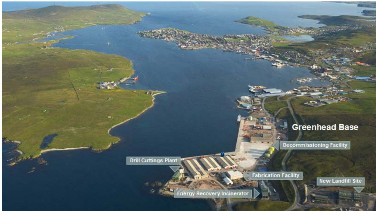
Figure 20 Port infrastructure built to service the Shetland Gas Project (photo: http://www.shetlanddecommissioning.com/decommissioning-services )
